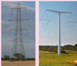
Lattice steel pylon T-pylon
